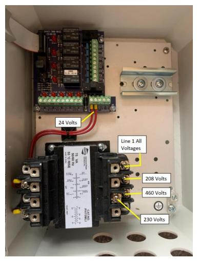
Figure 4-7: Input Wiring
